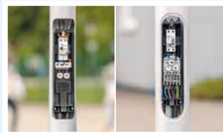
HSW technology in the mast of a street lamp
